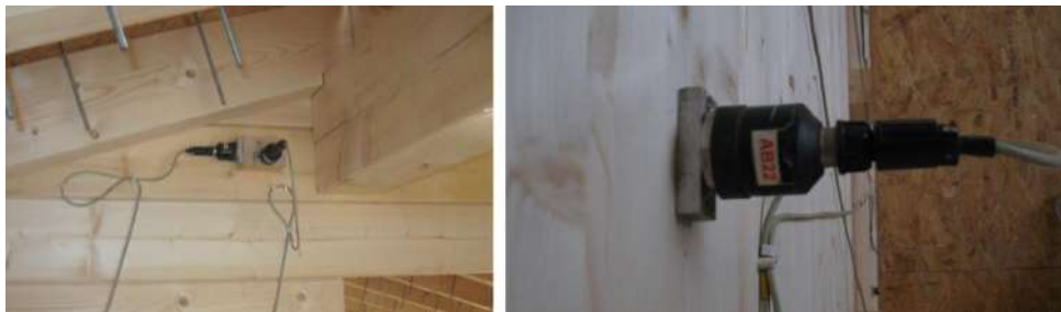
Figure 3.15: Accelerometers placed on interior wall (left) and close-up of an accelerometer (right)
